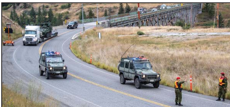
Cpl Cornfield of 12 MP Flt Comox and Cpl Bennett of 1 MP Pl Edmonton conduct traffic control in the Fraser River Valley to allow a flatbed transporting a LAV to have full access of the bridge.
