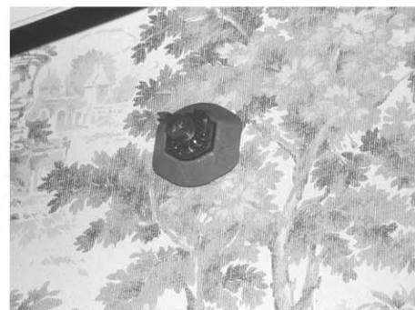
Figure 6. Sprinkler installed to blend with architectural wood finishes.
