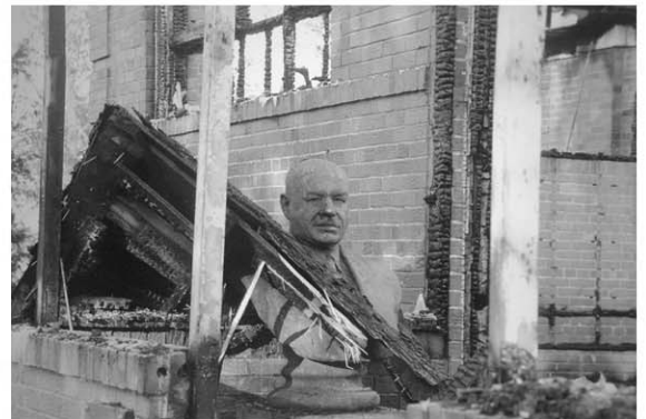
Figure 1. Aftermath of the fire at the Taras H. Shevchenko Museum, Oakville, Ontario.
