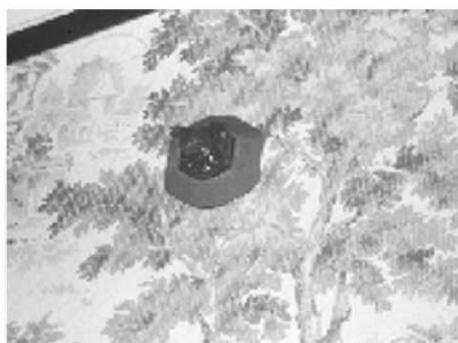
Figure 3. Sidewall sprinkler.
