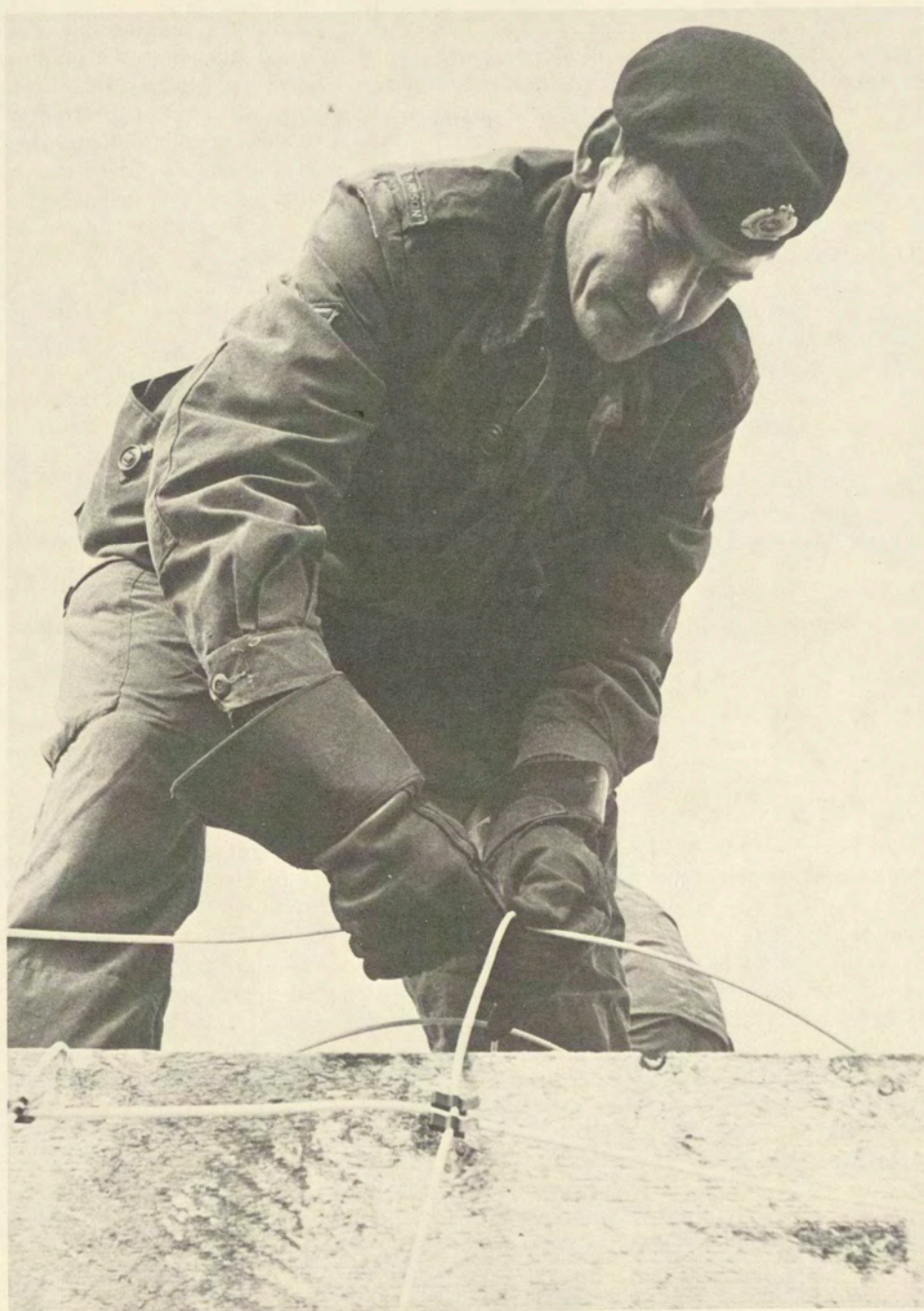
Demolition: a sapper in his element, preparing to make a loud bang
