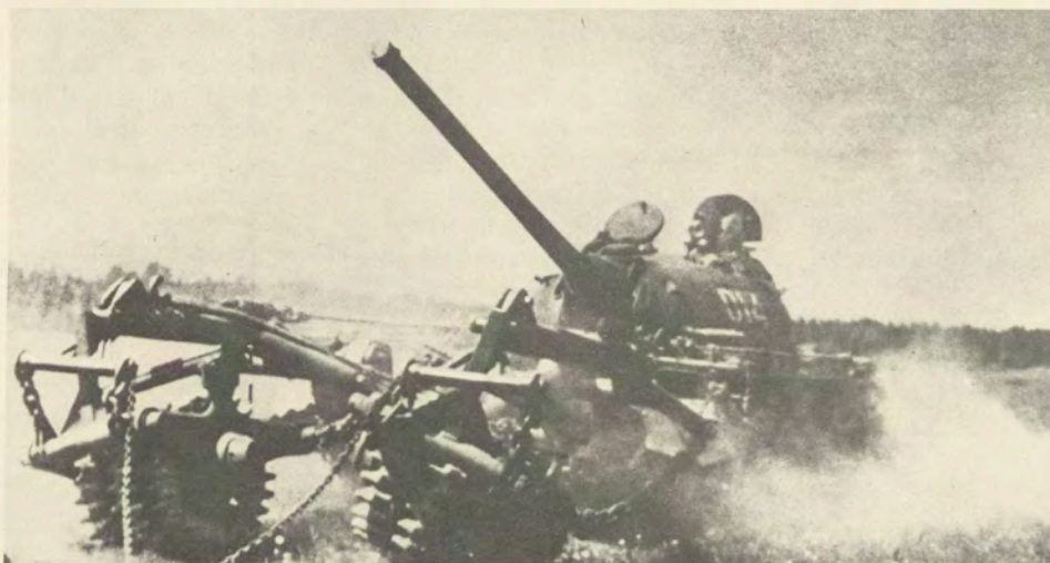
T72 equipped with KMT5 mine-plough
