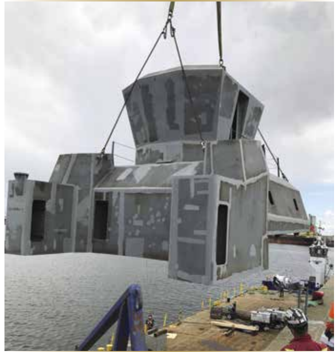
Figure 4. Superstructure assembled at the Industries Océan facility in Québec City is moved out of the construction hall for water transport 120 km down the St. Lawrence River to the Isle-aux-Coudres shipyard.
