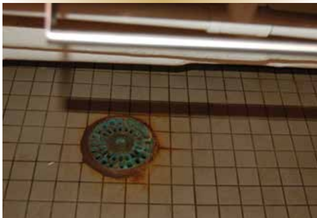
Figure 9. The problem with using dissimilar metals at connection interfaces.
