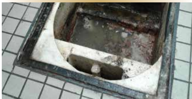
Figure 7. Galley grease trap coating breach and corrosion.
