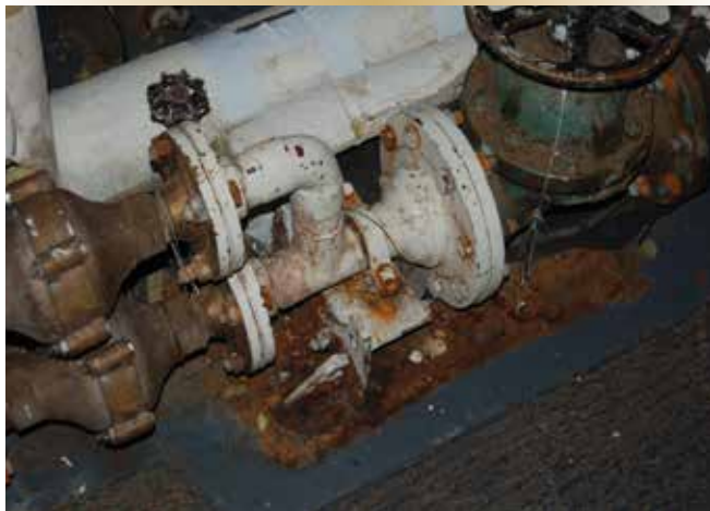
Figure 9. The problem with using dissimilar metals at connection interfaces.
