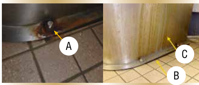
Figure 8. Corrosion on stainless-steel toilets.
