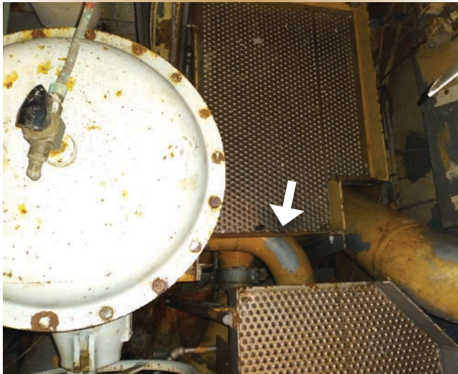
Figure 5. The auxiliary seawater circulation (ASWC) system supply in the after engine room.
