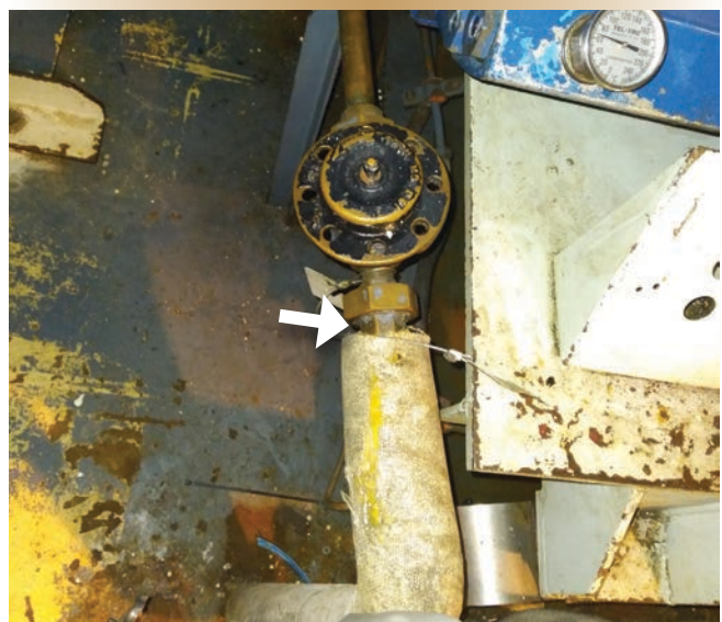
Figure 4. Flex line to the chilled-water return main.
