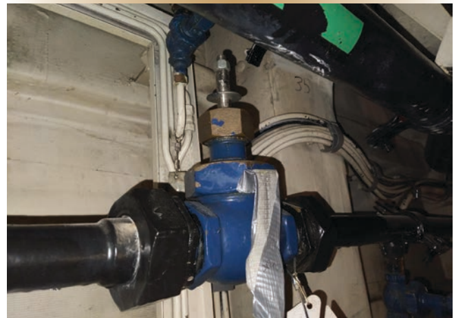
Figure 1. Screw-down non-return valve aboard a Halifax -class frigate.
