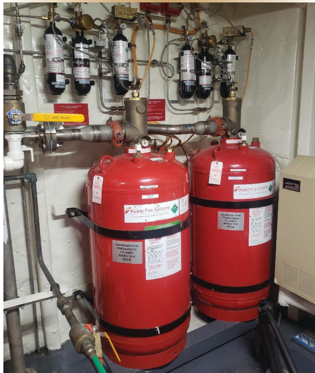
Figure 1. Novec 1230 arrangement on board HMCS Harry DeWolf for the port/starboard LV (low-voltage) spaces.
