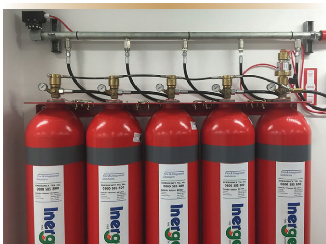
Figure 2. A typical IG-55 installation arrangement, similar to Halon 1301.
