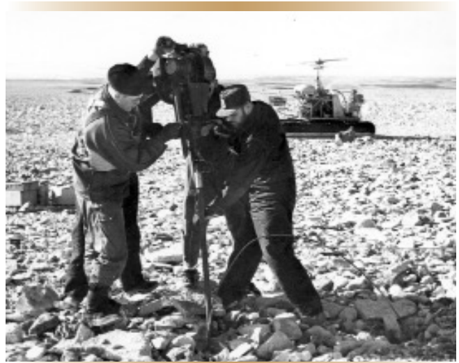
Lt. (P) John A. MacNeil & unidentified crew struggle with a gas-powered drill to set anchor bolts for a shore beacon.
