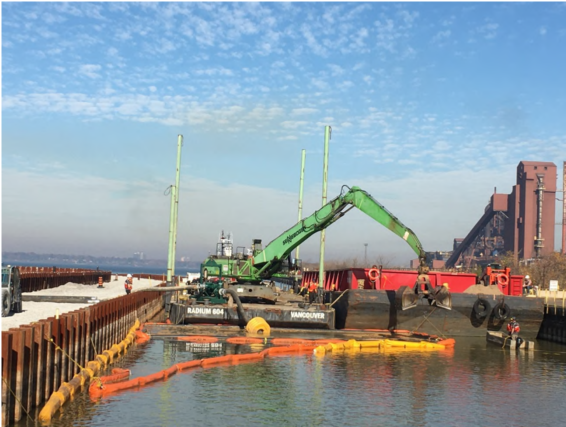
Figure CS4-7: Placement of the sand in the Stelco channel as part of the cap. (courtesy of Riggs Engineering)
