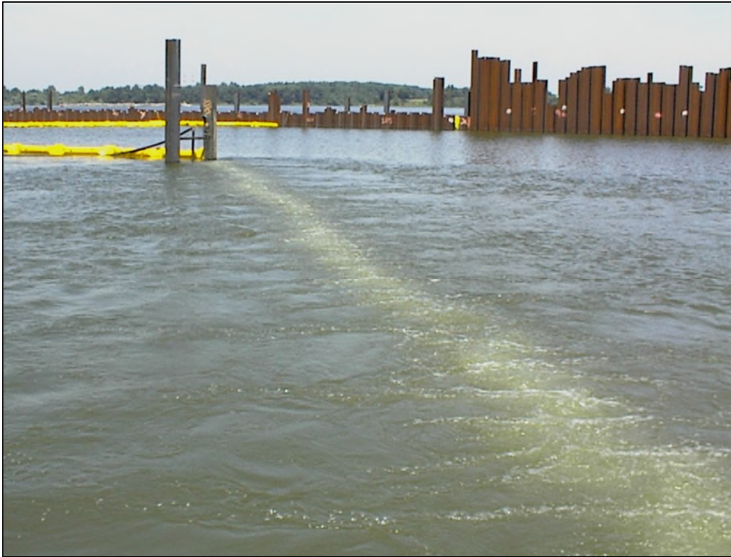
Figure 3-15: Bubble curtain deployment (courtesy of ECCC).
