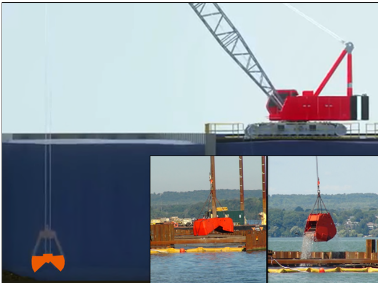
Figure 3-2: Mechanical dredge bucket deployment from a crane (courtesy of ECCC).
