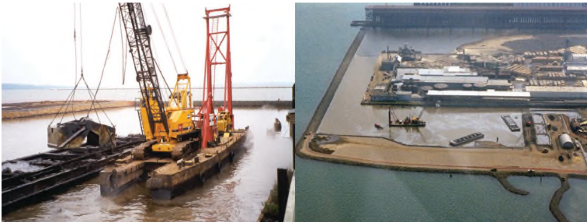
Figure CS1-4: (left) Dredging contaminated sediment using a Cable Arm clamshell environmental bucket and placement on a scow and (right) an overview of sediment handling, dewatering and the temporary storage area (courtesy of ECCC).
