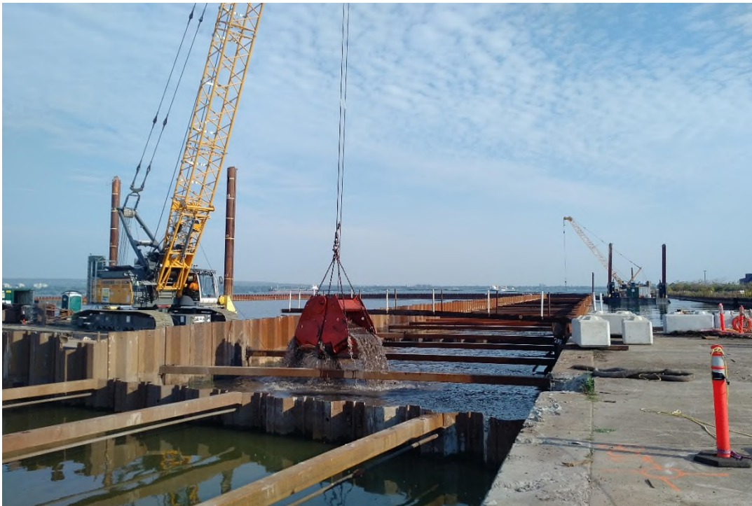
Figure CS4-5: Mechanical dredging was used to remove contaminated sediment from between the double walls of the ECF (courtesy of Riggs Engineering).
