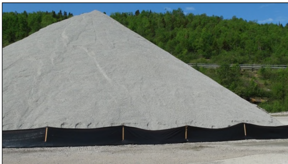
Figure CS2-5: Silt fences around the stockpiled sand (Capping material) (courtesy of ECCC).
