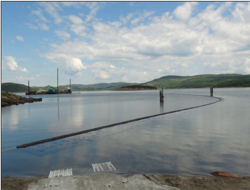
Figure CS2-4: Silt Curtains around near-shore habitats to protect fish habitat (courtesy of ECCC).
