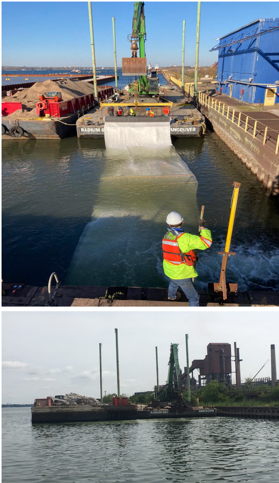
Figure CS4-8: Placement of the reactive core mat (top) and Erosion control (Bottom). (courtesy of Riggs Engineering)
