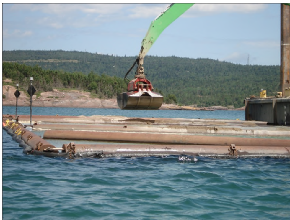
Figure 5-10: Capping using a mechanical clamshell (courtesy of ECCC).
