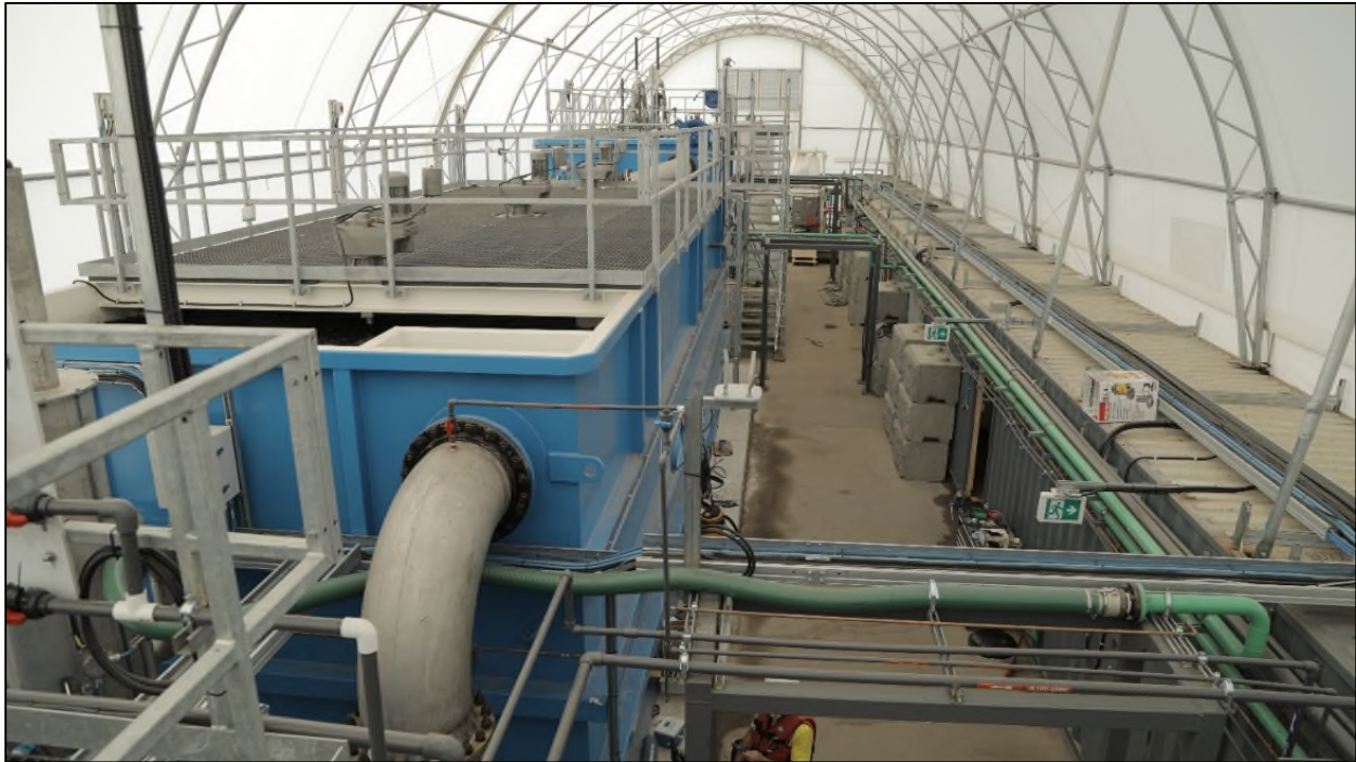
Figure 3-18: Settling cells in a water treatment system of the Randle Reef Sediment Remediation Project (courtesy of ECCC).
