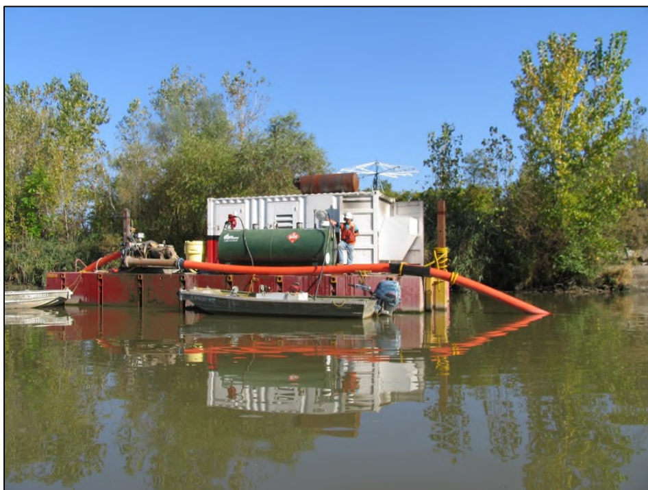
Figure 3-10: Booster pump configuration (courtesy of ECCC).
