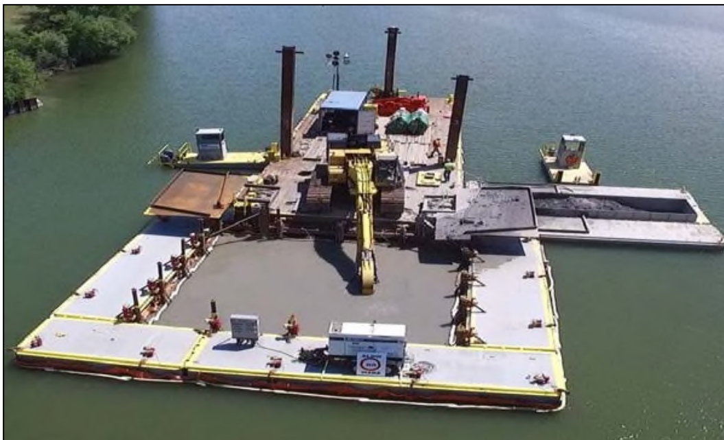
Figure 3-16: Derrick barge with attached moon pool and drip pans in use (M. Roberts, A. Corbin, P. Doody, T. Peters, and C. Robinson 2017).
