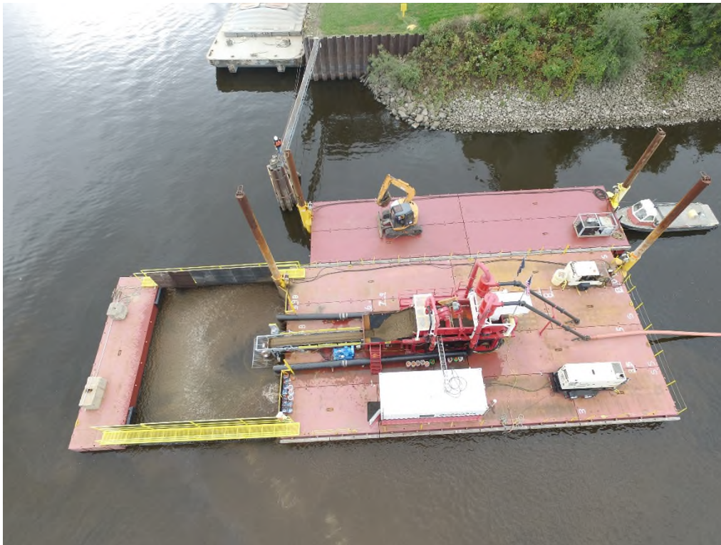
Figure 5-11: Spreader used for capping at the Fox River site, Wisconsin (courtesy of J.F. Brennan Company, Inc.).
