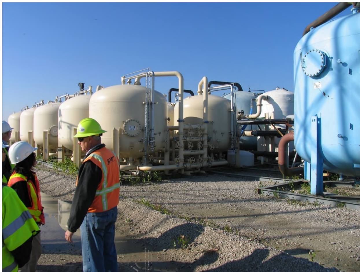
Figure 3-19: Sand filtration and activated carbon vessels in a water treatment plant (courtesy of ECCC).
