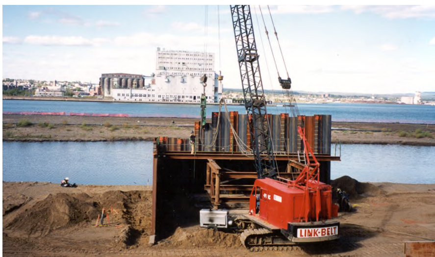
Figure CS1-6: Installation of Waterloo Sheet Pile Wall Barrier®(courtesy of ECCC).
