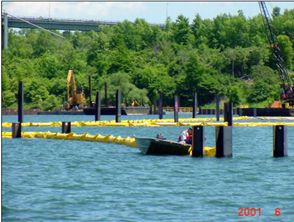
Figure 3-12: Silt curtain deployment (courtesy of ECCC).
