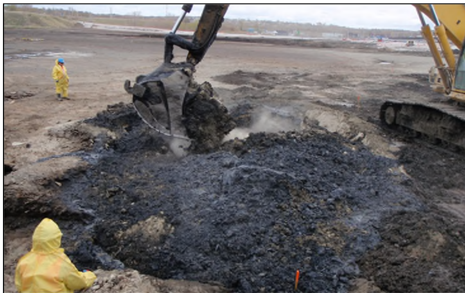
Figure 7-3: Solidifying sediment in the dry at the Sydney tar ponds (courtesy of Sydney Tar Ponds Agency).
