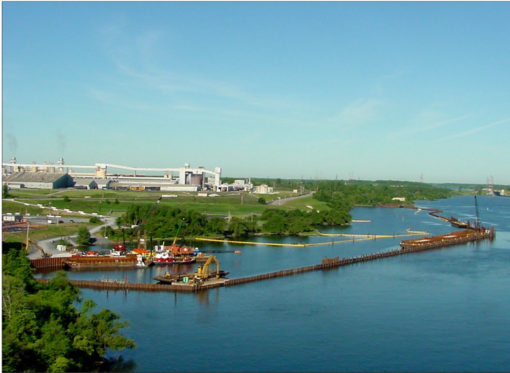
Figure 3-11: Temporary sheet pile containment (courtesy of ECCC).
