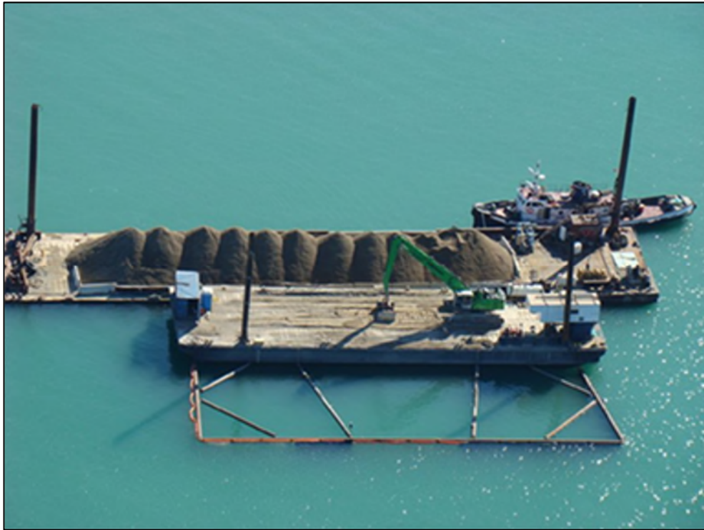
Figure CS2-3: A floating silt curtain box around the placement cell to minimize movement of fines (courtesy of Pacific Productions).
