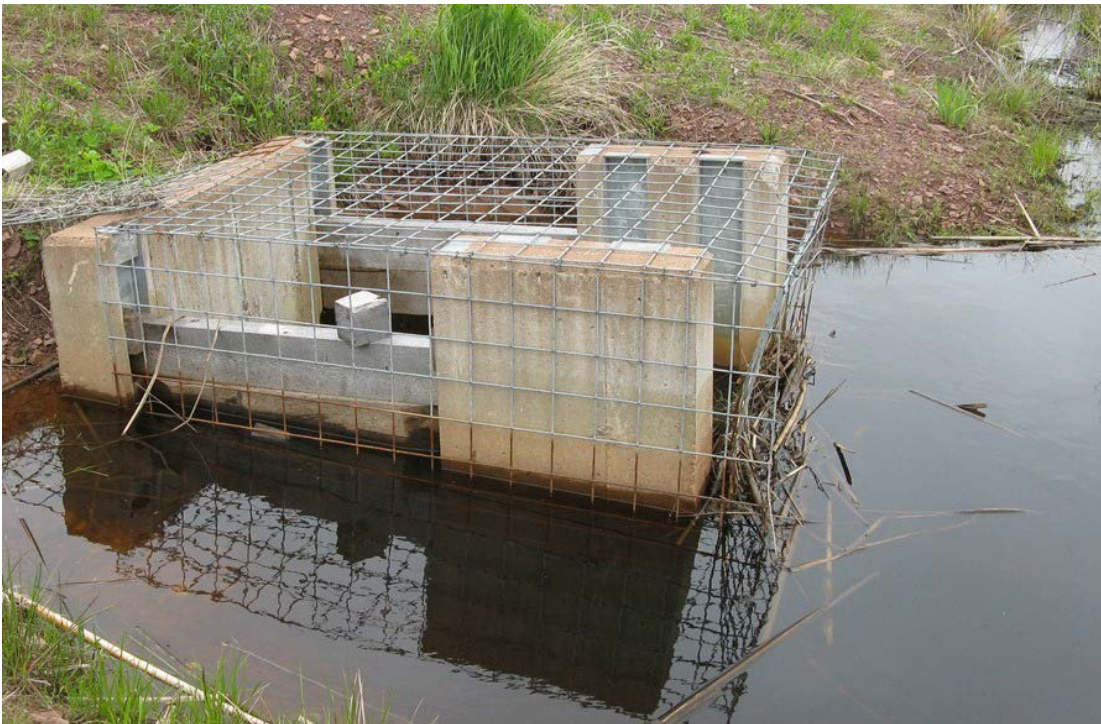
Figure 15: Example of a typical control structure used to regulate water levels within an impoundment. A wire cage is applied to reduce plugging from beaver activity. Photo: C. MacKinnon © Environment and Climate Change Canada, 2013
