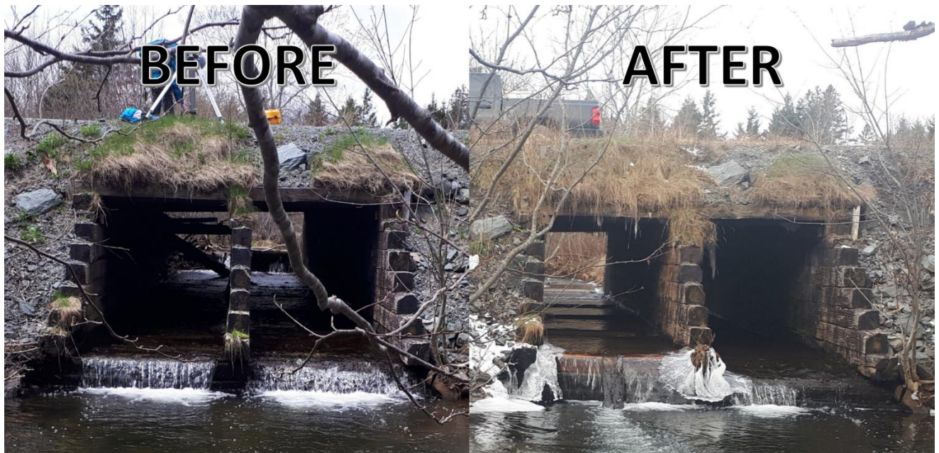
Dry Brook fish passage improvement project where wooden baffles, a low flow barrier, and an outflow chute were installed on a double wooden box culvert.
