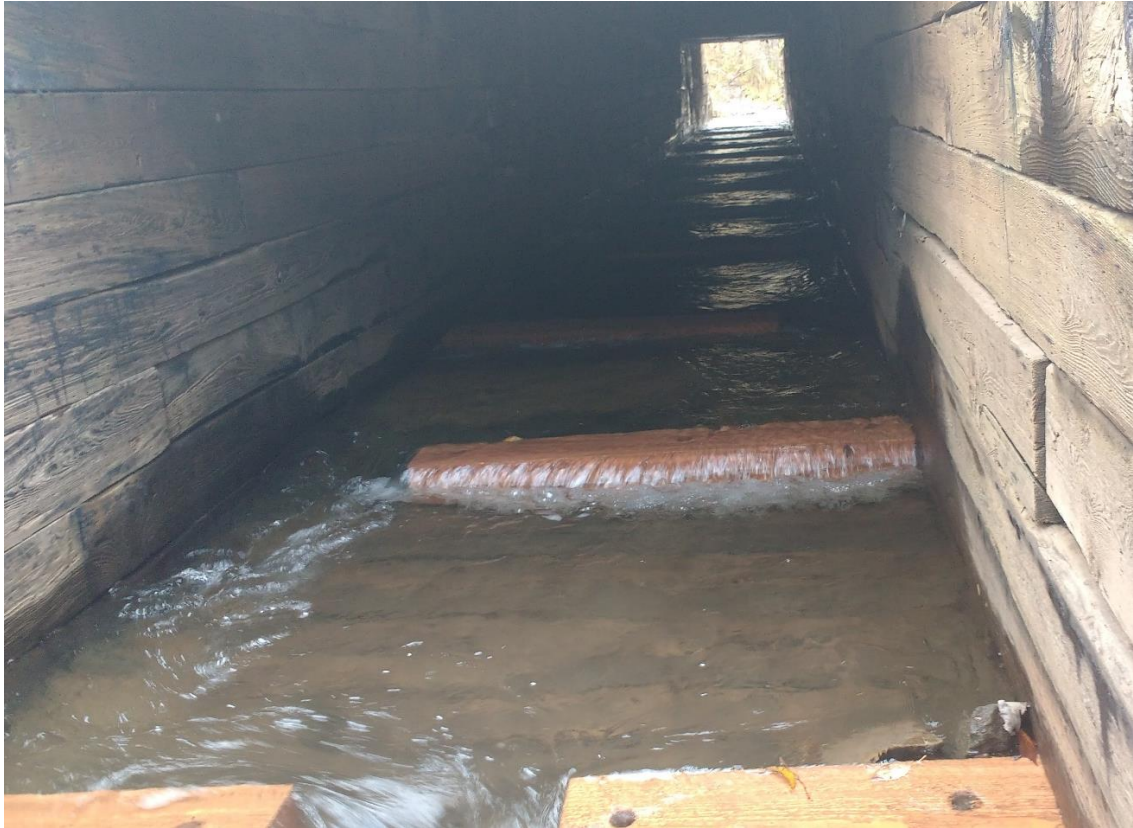
Moore Brook fish passage improvement project where hemlock 10"x10" timbers were installed as baffles to increase depth and decrease velocities.
