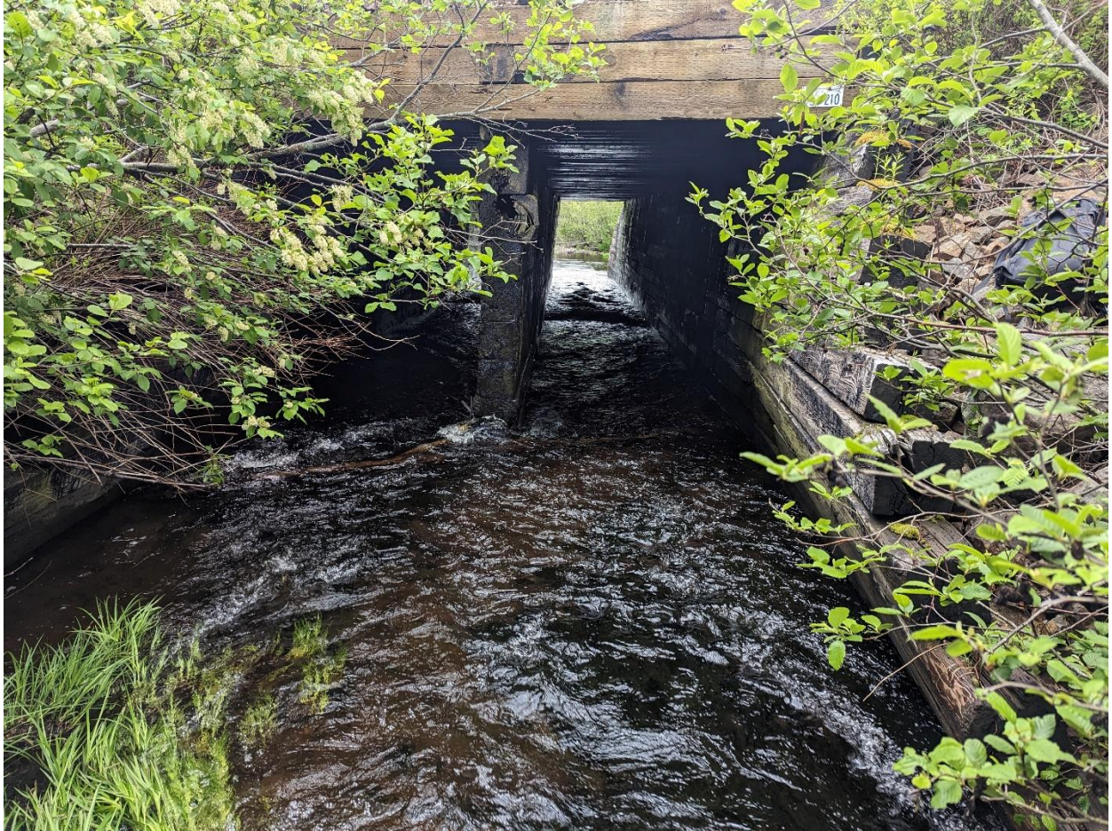
Looking at culvert inflow from upstream
