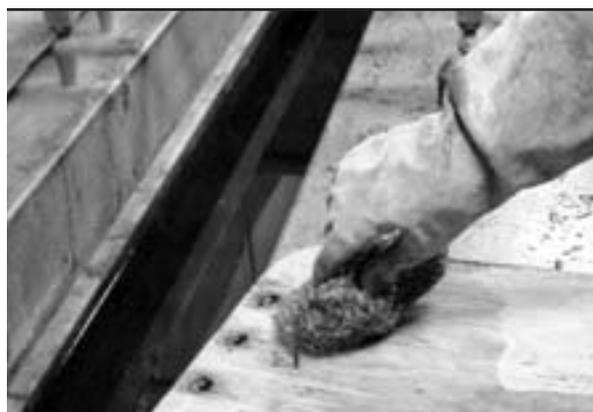
Wipe the stripped surface with a damp steel wool pad instead of hosing it down.
