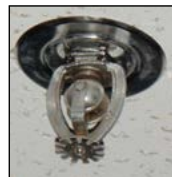
Showerhead of fire extinguishing system
