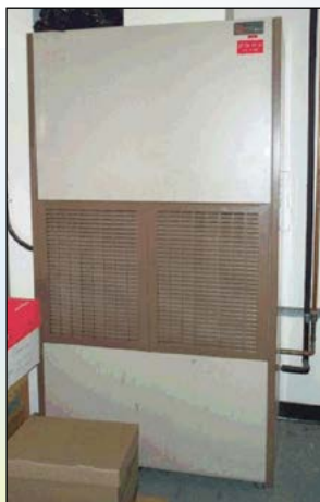
Air conditioning evaporator
