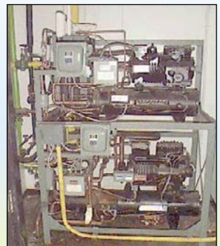
Walk-in refrigerator compressors
