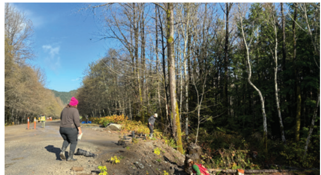
The Restoration Centre of Expertise assisted the Squamish Watershed Society in planting new vegetation following culvert installation. (Photo by Sydney Bryce, DFO)
