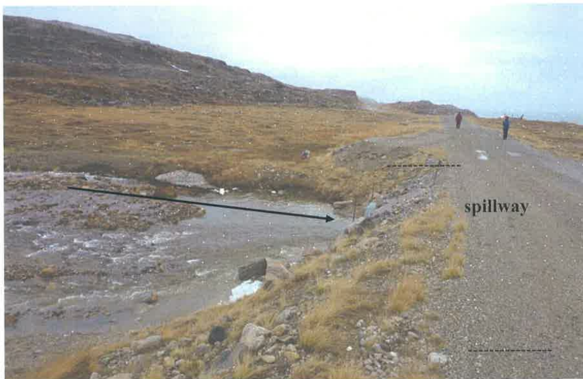
Photo 8. Secondary road and stream crossing with two culverts. Possible location of spillway.
