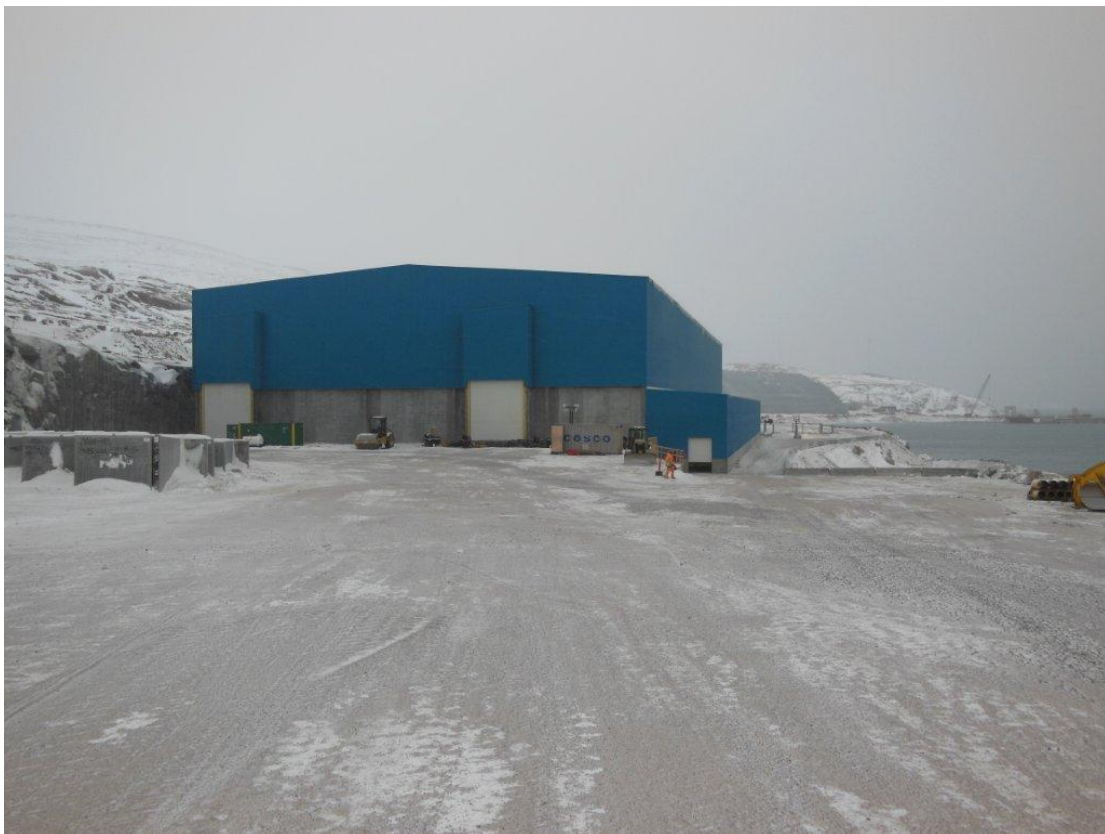
Storage hall, Q1 site (november 2012)
