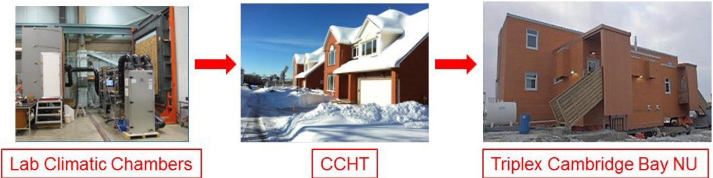
Figure 1: Facilities used in this study.
