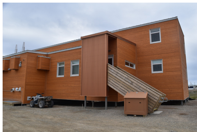
Figure 1: Triplex residence at the CHARS where the greywater system was installed.
