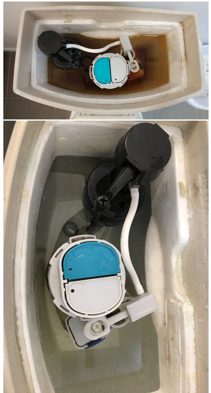
Figure 8: Toilet tank before (top) and after cleaning and flushing with treated greywater (bottom).
