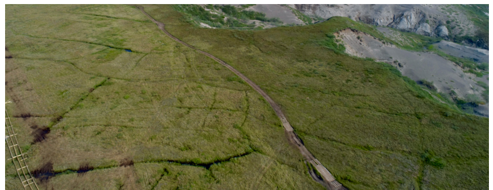
This aerial photo (above) shows the new Kugluk Territorial Park ATV trail under construction in 2019. Ice wedges, a feature of permafrost, are visible. The permafrost soil sample (upper right), collected along the ATV trail, has high ice content: POLAR
