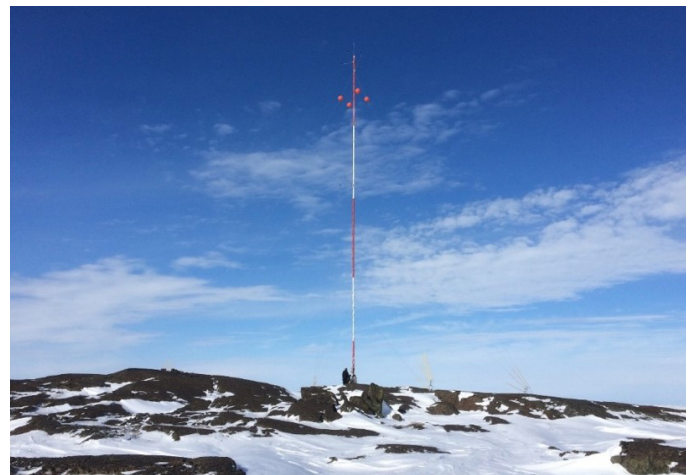
Wind tower positioning in Sanikiluaq, NU: QBDC.
