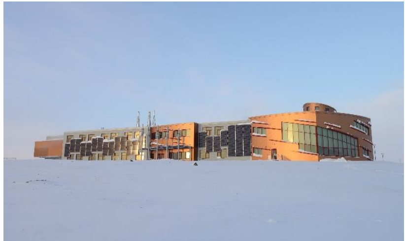
The Main Research Building of the Canadian High Arctic Research Station (CHARS) includes research labs, centres for technology development and knowledge sharing, office space, and spaces for teaching, training, and community engagement. Photo: A. Fradkin
