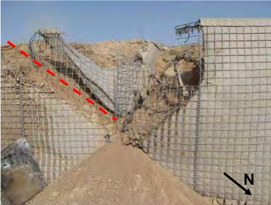
Photo 3: Damaged barrier showing main rotor blade strike
