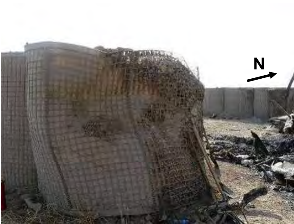
Photo 2: Damaged barrier showing side of aircraft impact
