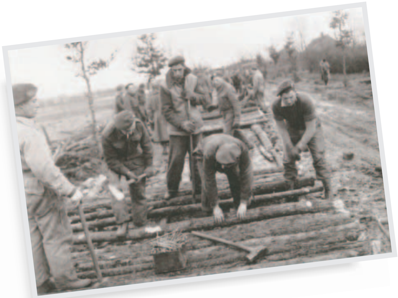
Sappers also had to maintain all types of roads, and adapted 19th-century techniques when necessary. (PA 140645)
