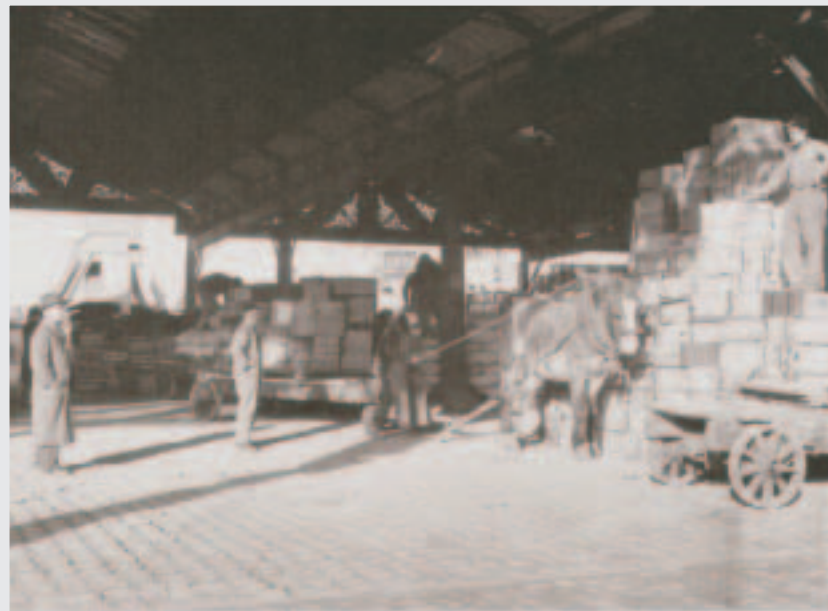
.. and once the approaches were cleared, the ships were unloaded quickly, using all available technology. (PA 192024)
