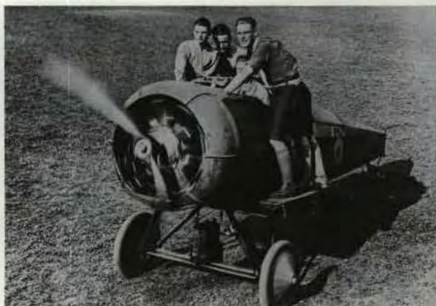
Instruction in the intricacies of the magneto and engine ignition was given on wingless (and sometimes tailless) machines known as 'penguins.' (AH 518)
