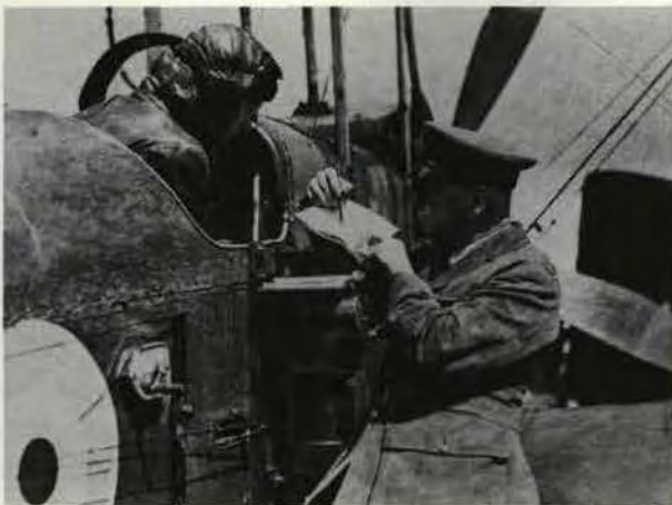
A photographic officer points out to the pilot of a BE12 the areas to be photographed. The map is resting on the aerial camera. (Q 12288)
