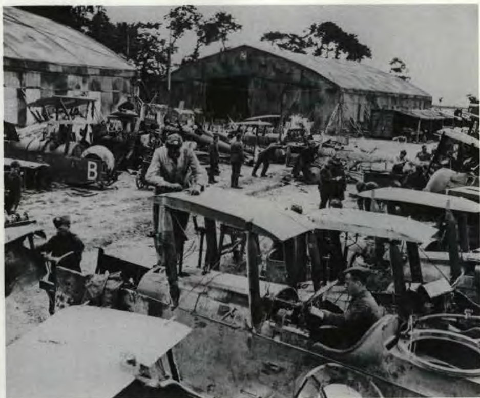
An RFC aircraft repair park. The machine in the foreground, with an instrument mechanic sitting in the pilot's cockpit, seems to be a DH9. Other aircraft include Sopwith Camels, an SE5a, and a DH4. (AH 433)
