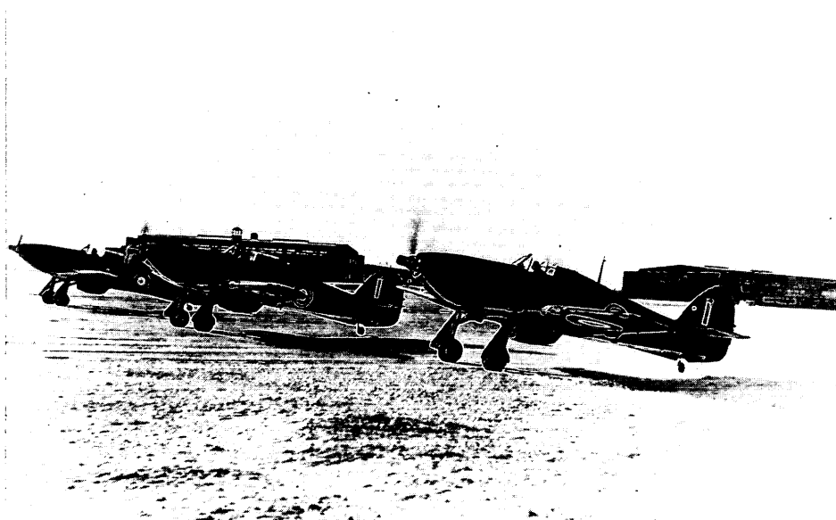
Air defence for Newfoundland: Hawker Hurricanes of 127 (F) Squadron, Gander, December 1942. Canadian-built Hurricanes were distinguished by large American propellers, which could not be capped by the spinners characteristic of British Hurricanes. (PL 14155)
