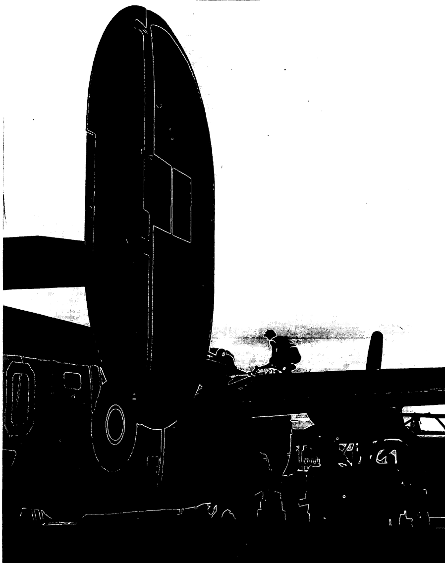
Refuelling a 10 (BR) Squadron Liberator at Gander in the summer of 1943. This particular aircraft has had most of its secondary armament removed in order to conserve weight and thereby increase range. (PL 21169)
