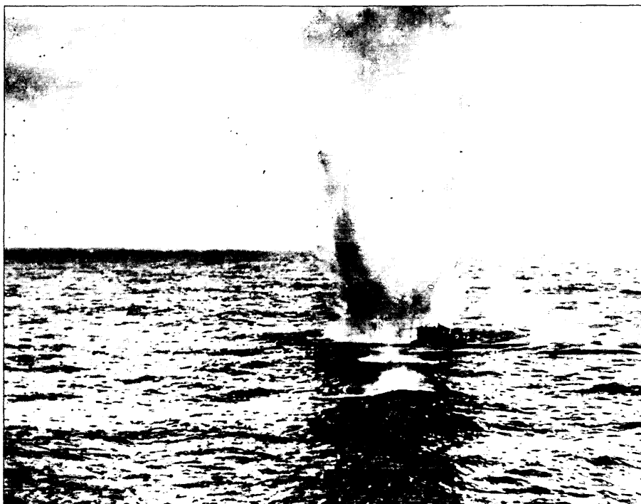
The destruction of U-342 by Flying Officer T.C. Cooke of 162 (BR) Squadron on 17 April 1944. The plume of the first depth charge has reached its apex, the dome of the second has just begun to rise, while the entry splash from the third charge is visible in the foreground. (PL 25259)
