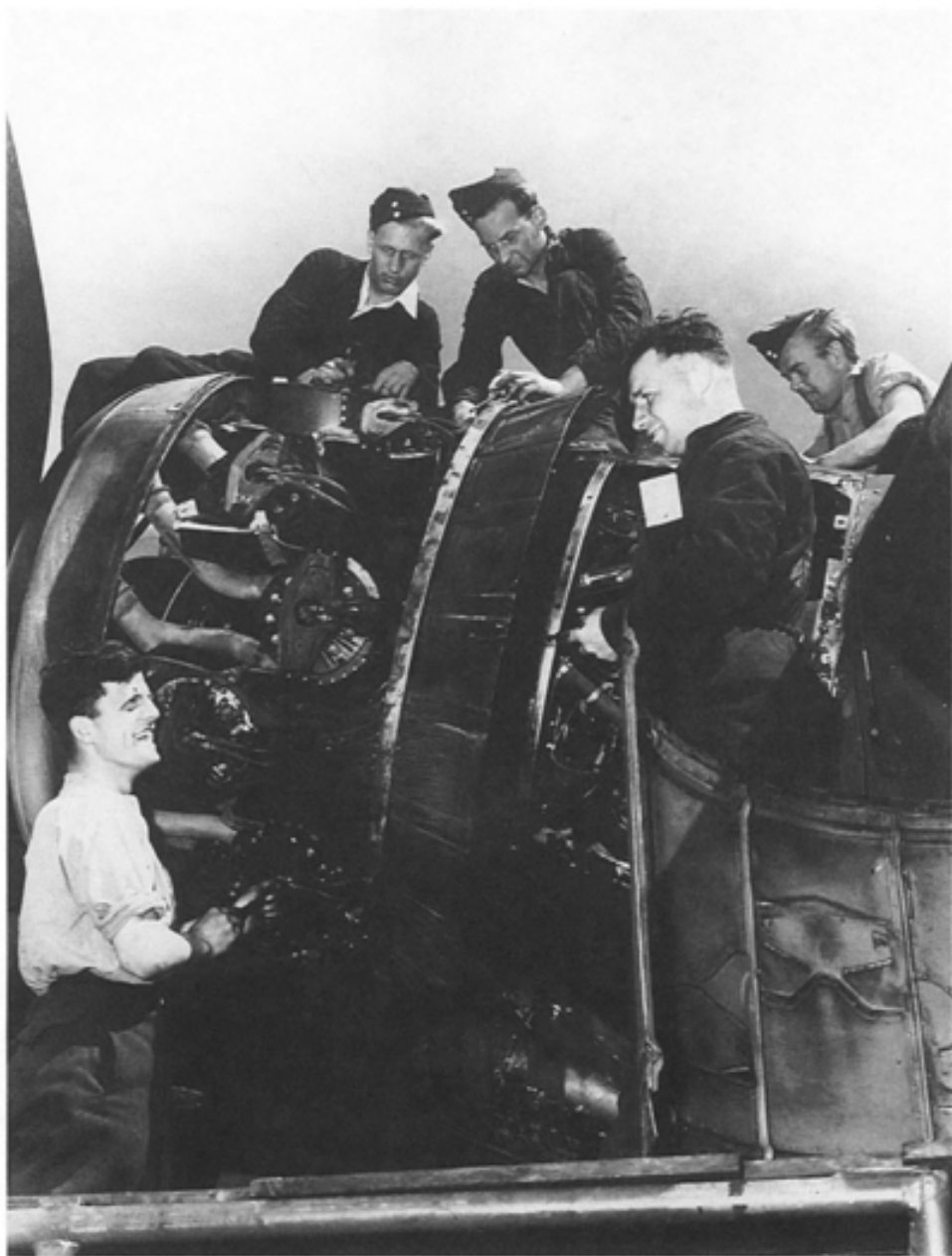
Fitters of No 420 Squadron work on the Hercules engine of a Halifax in the summer of 1944. (PL 30746)
