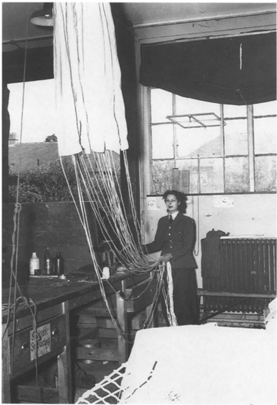
A parachute rigger with an RCAF squadron in the delicate task of straightening the cords of the parachute before repacking. (PL 4915)
