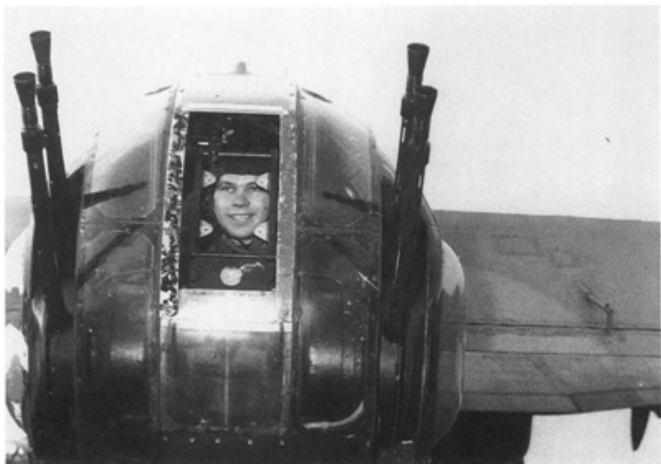
Until the very end of the war the main rear defence provided for heavy bombers was a tail turret mounting four .303-inch machine guns. Although the installation was reliable and the guns could maintain a very high rate and volume of fire, they lacked range and destructive power. (PL 22001)
