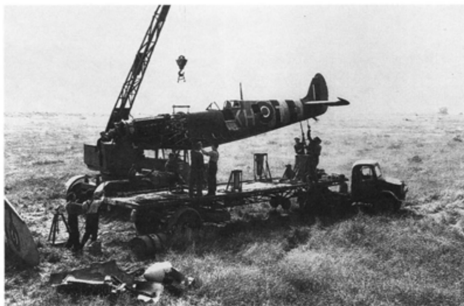
A Repair and Salvage crew recovers a No 403 Squadron Spitfire in the field. (PL 31115)
