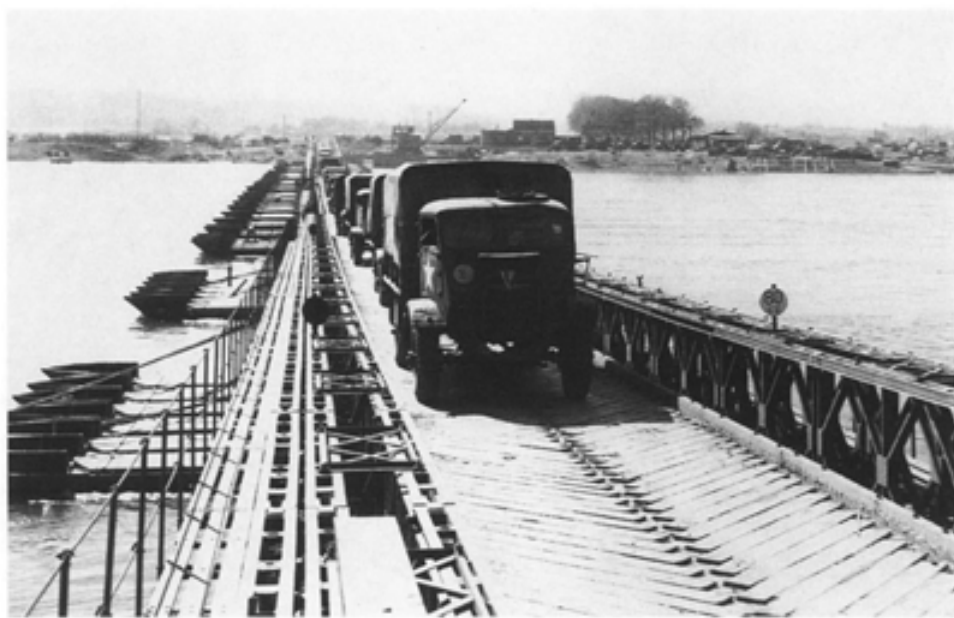
A No 143 Wing convoy crosses the Rhine on a Class 80 Double-Single Pontoon Bailey Bridge in April 1945. (PL 44575)
