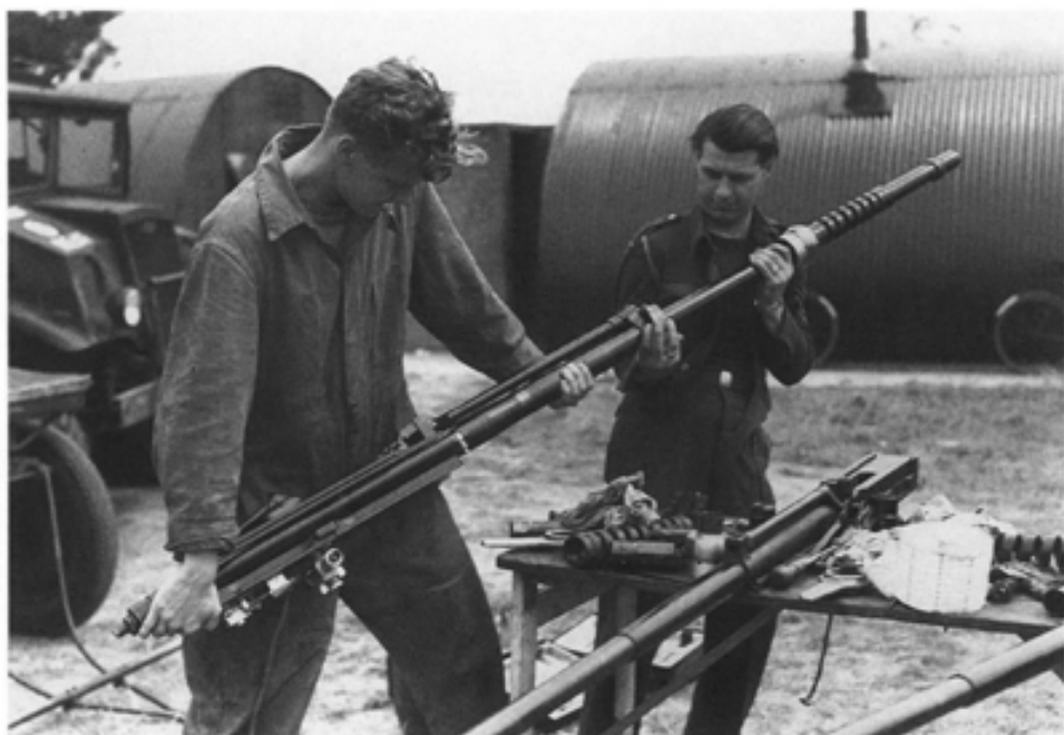
No 409 Squadron armourers work on the cannons of a Mosquito in the summer of 1944. (PL 31818)
