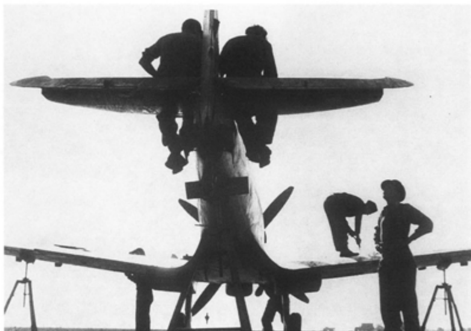
With levelling jacks supporting the wings and rear fuselage and a plumb bob hanging from the machine's nose, the guns of a Spitfire are harmonized. (PL 18516)
