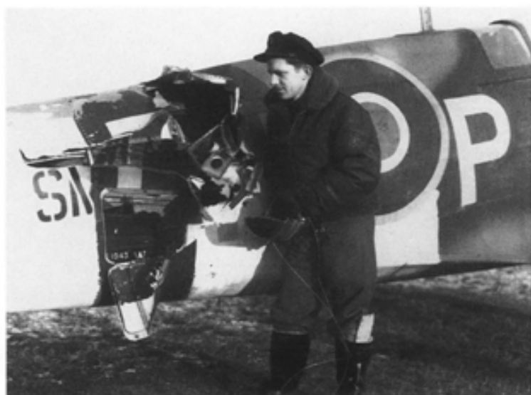
Flak damage sustained by a No 416 Squadron Spitfire on Christmas Eve, 1944. (PL 41349)
