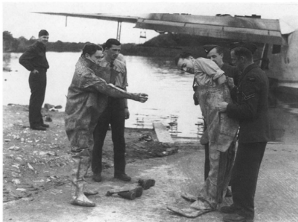
In order to work in the frigid waters of Lough Erne at Castle Archdale, Northern Ireland, mechanics had to put on rubberized wading suits before making their repairs. (PL 40986)
