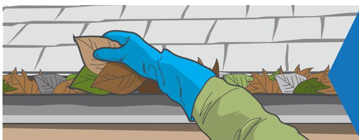
Clear leaves from eavestroughs, downspouts, and drains.
